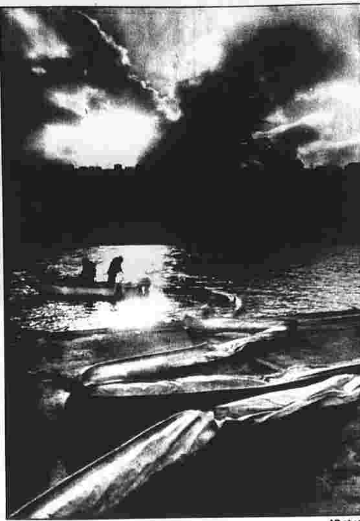
LIGHT CLEANING — Workers drag a boom Monday into the Monongahela River as part of the cleanup of the million-gallon spill of diesel fuel in Pittsburgh.
